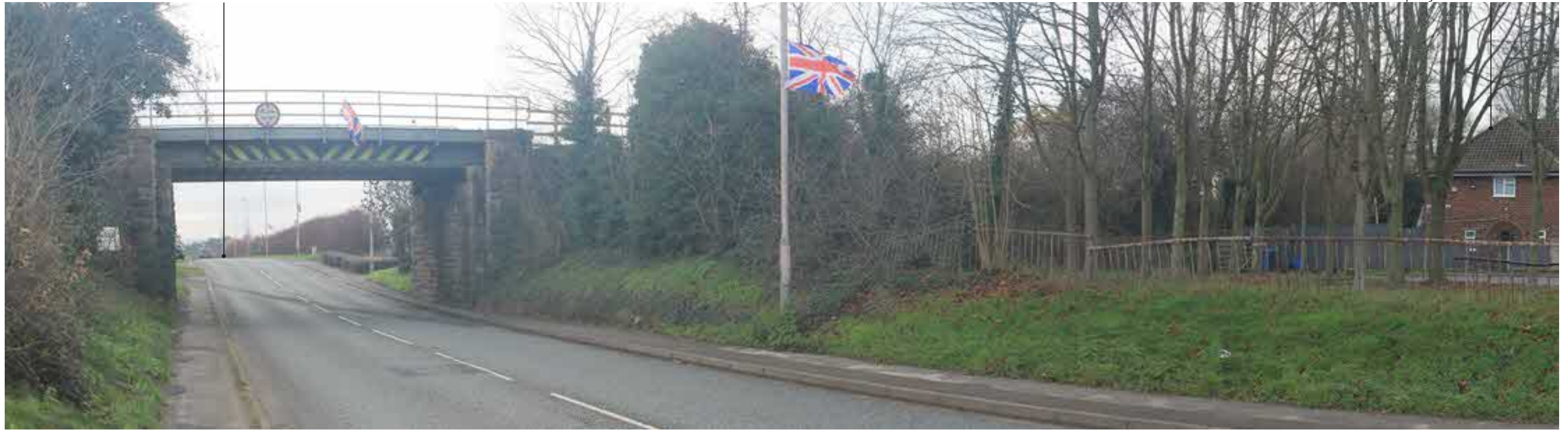
Photograph 12 View from Mansfield Road, looking south west towards the Site
