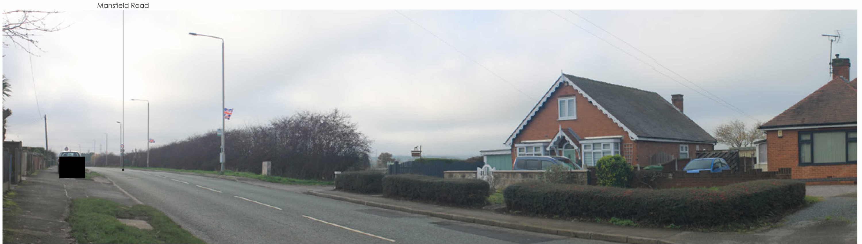
Photograph 13 View from Mansfield Road, looking south west towards the Site
