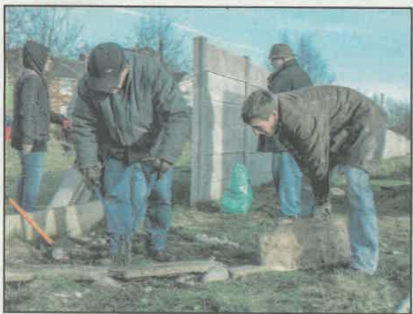
Volunteers working together to repair the damage.
